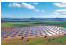
Profitable solar radiation: In October GILDEMEISTER has finished a solar park with 90 “SunCarriers” in Spain (Pozohondo).
